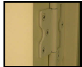
Hinge spacer installed.
