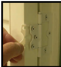
Insert hinge spacer.
